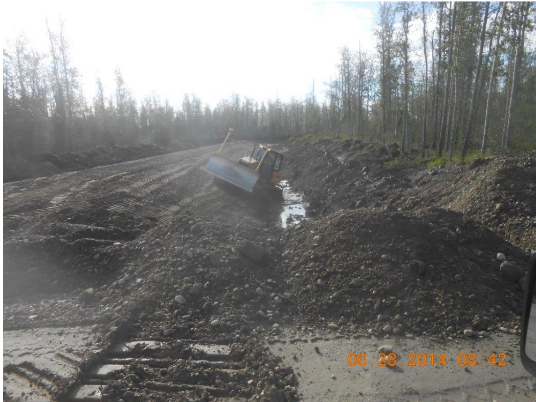
Spur Dike Construction
